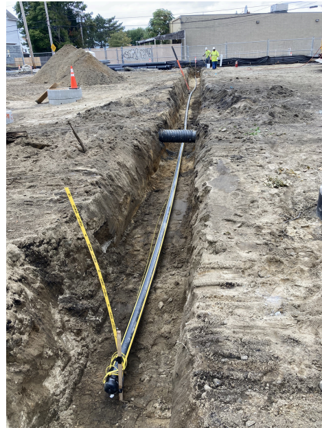
Gas line installation
